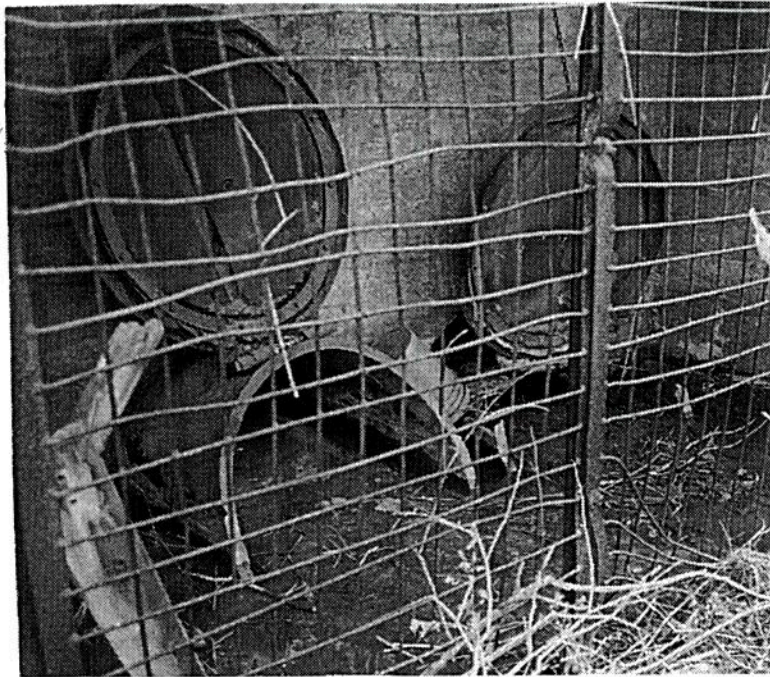
The two inlet pipes on the marsh side of the embankment
