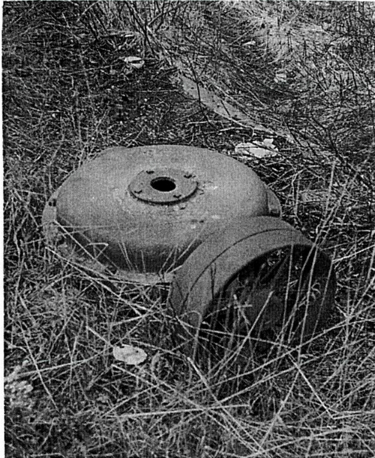
One of the original pumps with the pulley still attached
