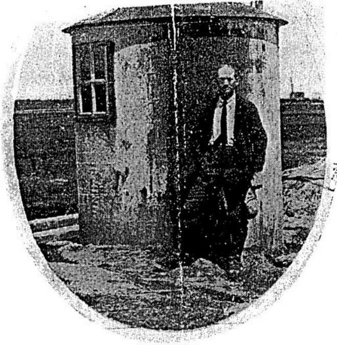
Prof Day Standing in front of the Bradford Scheme Pump House - 1929
